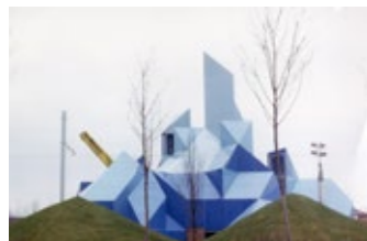
Under construction - Iain Bruce
